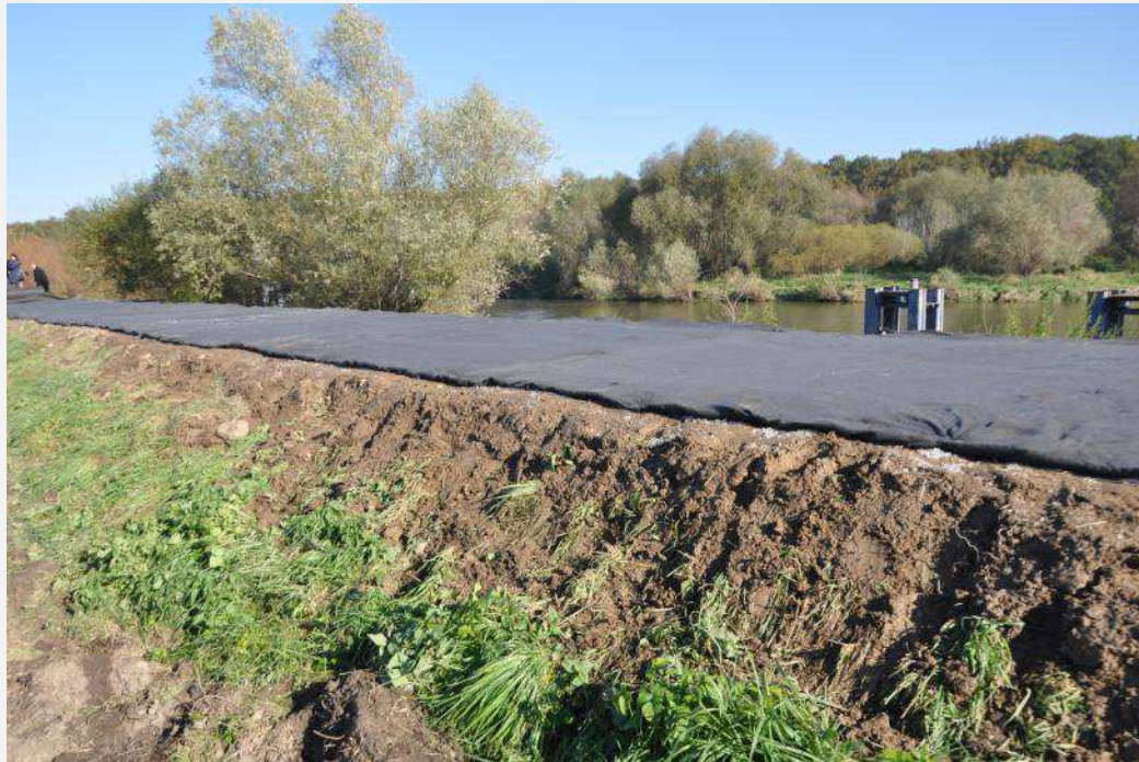
Water absorbing geocomposites during installation on the Odra River embankment
